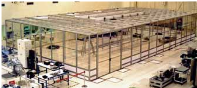
Modular cleanrooms as large as 5,000 square feet, and even larger, are often required for assembly lines, packaging operations and other environments.
