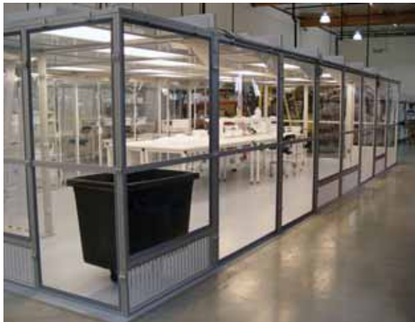
A well-organized cleanroom includes attention to process flow. Make sure furniture and equipment do not hinder air flow. Materials should come in one end and go out the other.
